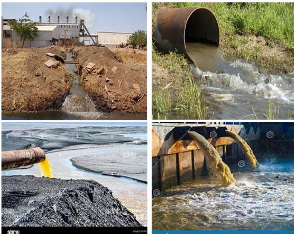
Figure 1. Different discharge sources of industrial wastewater in water bodies
